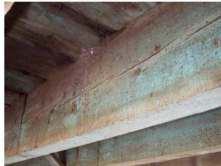
Fonte: BRIDGE INSPECTION MANUAL – NY'S DOT
