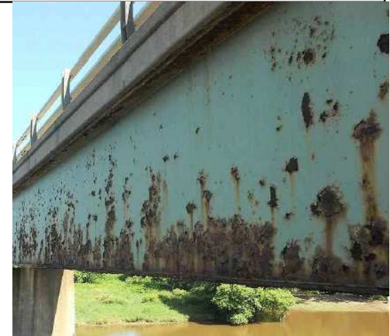
Fonte: BRIDGE INSPECTION MANUAL – NY'S DOT
