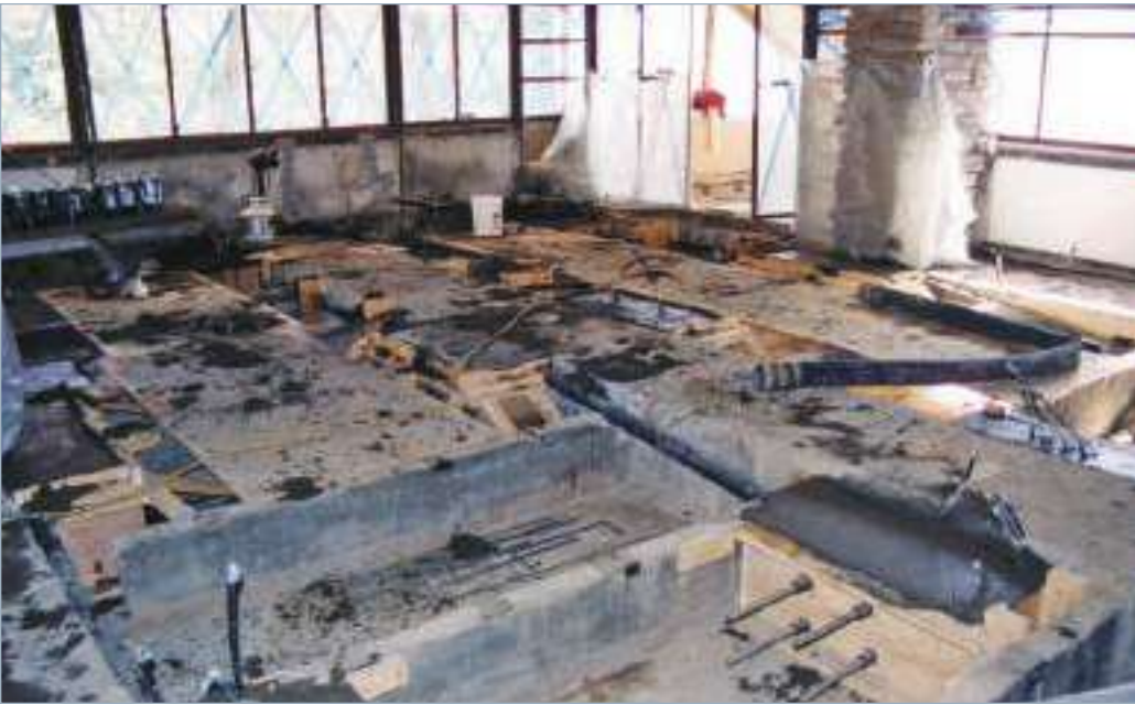
Living room floor reinstallation at Fallingwater, 2002, view of cable channel anchors following concrete pouring. This work was completed as part of an overall preservation effort to slow the deflection of the house's terraces. Structural monitoring of the terraces in 2013-2014 has proved the post tensioning cable installation beneath the living room floors a success. Photograph courtesy of Fallingwater and the Western Pennsylvania Conservancy.
