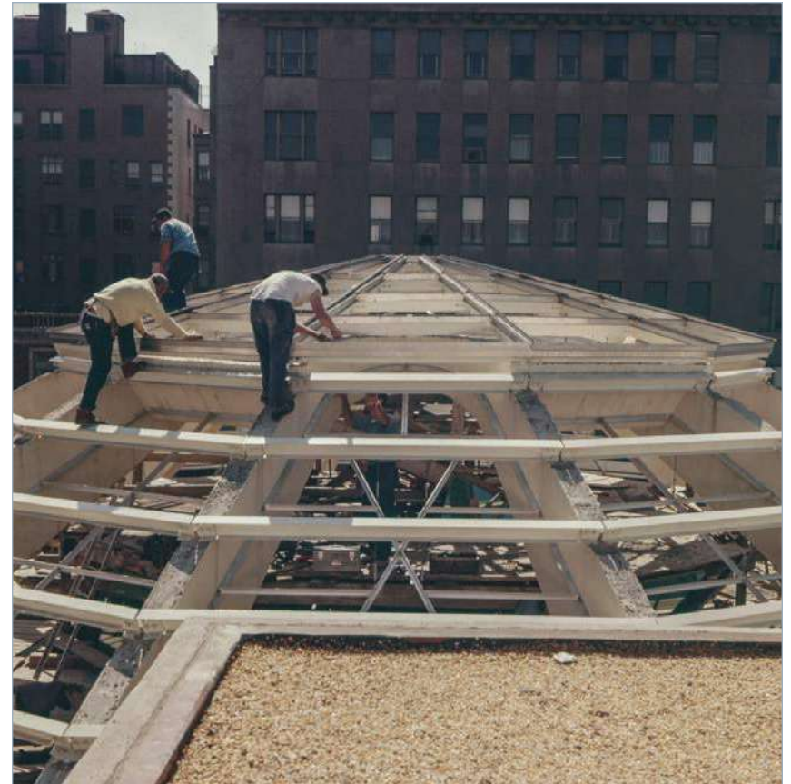
Solomon R. Guggenheim Museum, view of installation of skylight glass, ca. 1956 - 1957. Photograph by William Short. Courtesy of the Solomon R. Guggenheim Foundation.
