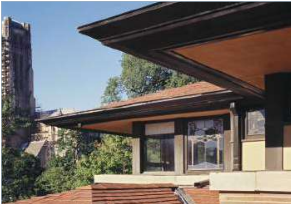
Frederick C. Robie House, view looking up from courtyard showing raked Roman brick and mortar detail of piers. Photograph courtesy of Frank Lloyd Wright Trust.
