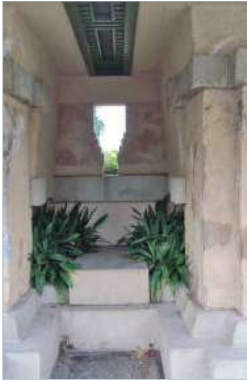
Preservation of the loggia near the entrance to Hollyhock House was completed to investigate surface cracks in the concrete stucco exterior as well as any possible structural problems. Once completed, the surface was repaired and plastered and covered with a coat of paint. Photograph by Jeffrey Herr, courtesy of Hollyhock House.
