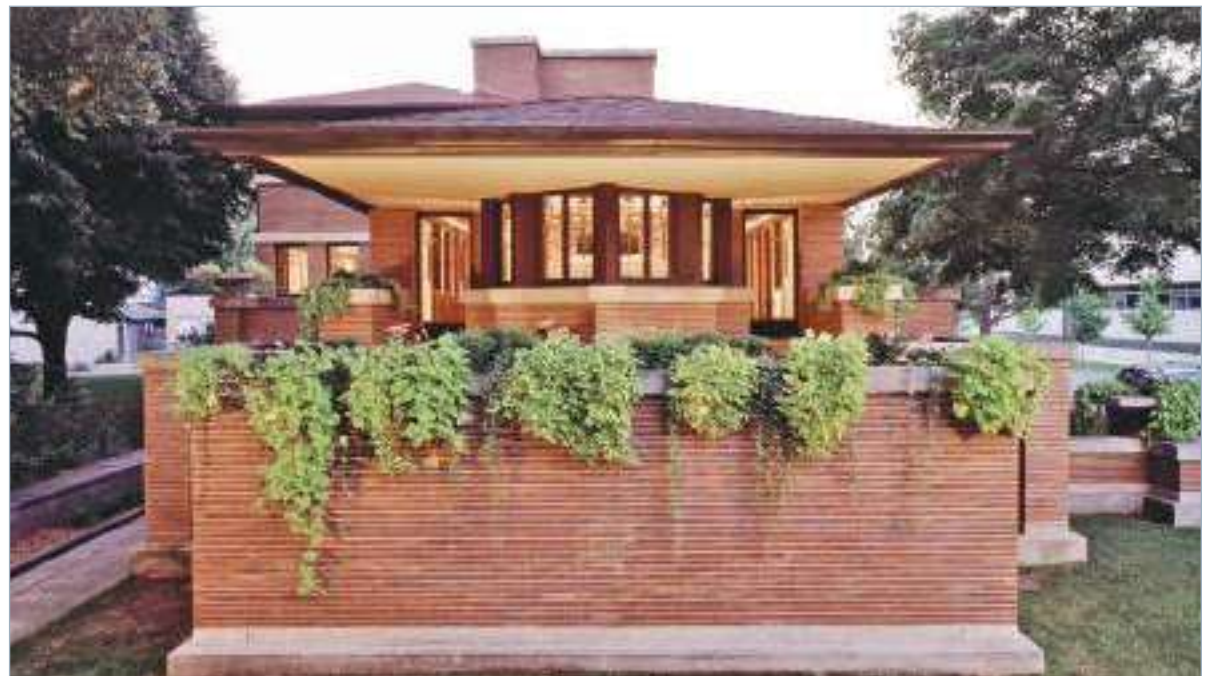
Frederick C. Robie House, view of the north elevation of the house showing porch and dramatic cantilever of roof over the north prow, concealed entrance to the house (left) and building-length balcony of main level (right).
