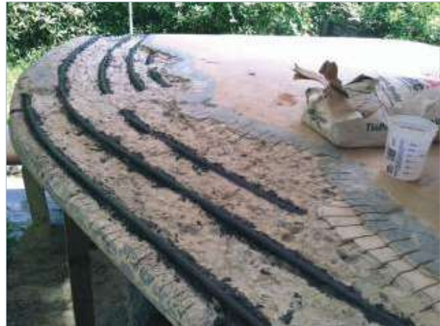
As part of ongoing preservation of Fallingwater, the concrete step canopy of the stairs leading from the main house to the guest house was repaired following cracking and material loss in June 2013. The work provided insight into the concentric arrangement of the canopy's reinforcing system, shown here after treatment with an anticorrosive agent. The concrete was reapplied and the rolled edges of the canopy formed by hand before applying the finish paint coat.
