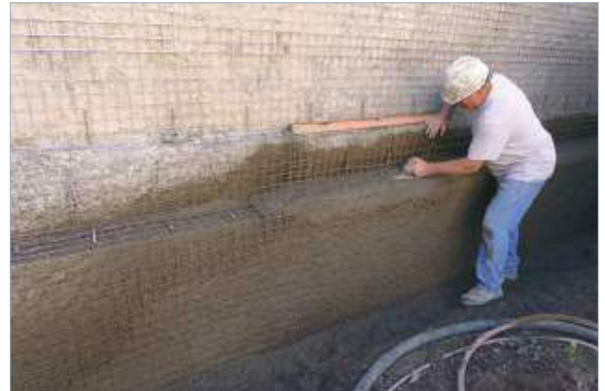
Unity Temple, application of concrete finish to exterior walls where it had been removed due to degradation.
