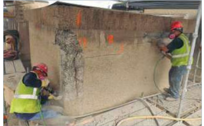
Unity Temple, removal of degraded exterior concrete finish during restoration of building's exterior to historic appearance.
