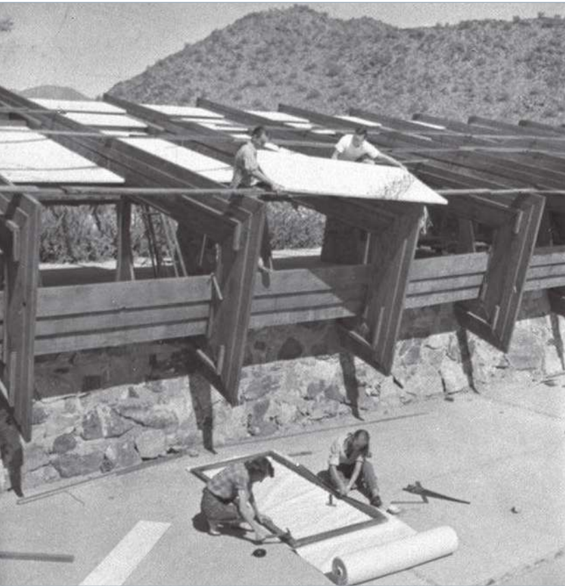
Taliesin West, view of drafting studio during canvas roof replacement, 1946.
