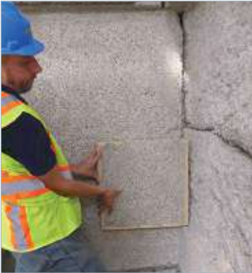
Unity Temple, sample of desired exterior concrete finish compared to existing conditions.
