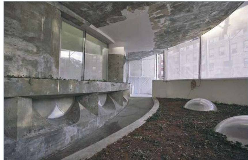
Façade with paint removed during preservation of the Solomon R. Guggenheim Museum, 2005. The preservation effort removed eleven layers of paint from the surface, resulting in a revelation that Wright's original pigment was a light-yellow "buff" shade, used only until the early 1960s. The color became more off-white or gray over time, and in the end, the museum was painted off-white, the hue most associated with the building's history. Photograph by David Heald, courtesy of the Solomon R. Guggenheim Foundation.
