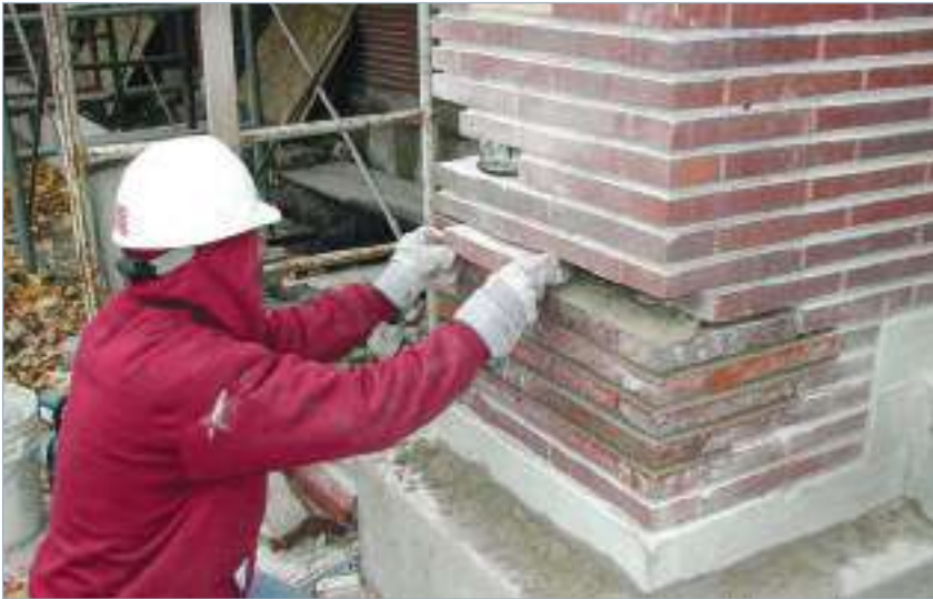
Installation of salvaged bricks on the south façade of the Frederick C. Robie House, November 2002. The replacement bricks were used in areas where missing and or severely damaged bricks were found, in this case on a pier on south façade of building.
