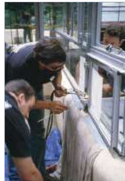
Steel window conservation along the exterior walls of the living room hatch at Fallingwater, September 2001. The steel sash conservation is ongoing, with each window and door frame monitored for corrosion. The paint layer is removed, the steel frames repaired, and an ultraviolet light-filtering glazing replaced.
