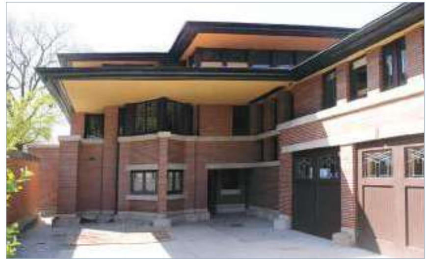
Frederick C. Robie House, view of south elevation showing main level's south porch and its cantilevered roof eaves, third floor bedroom level, and courtyard with staff quarters over former garage (now museum gift store).
