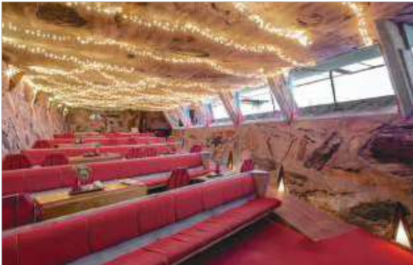
Taliesin West, view to the southeast of Cabaret Theater interior showing desert masonry wall and ceiling construction. Photograph by Andrew Pielage, courtesy of the photographer.
