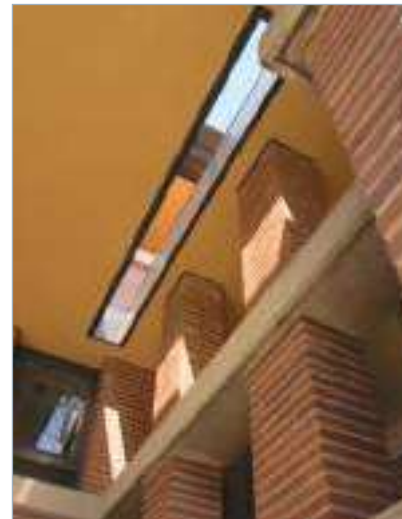
Frederick C. Robie House, view looking up from courtyard showing raked Roman brick and mortar detail of piers. Photograph courtesy of Frank Lloyd Wright Trust.
