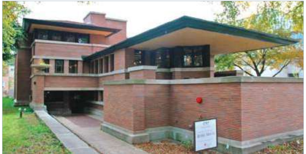
Frederick C. Robie House, view showing northeast corner of house with ground-level concealed entrance (left) and main level's northern prow and north porch with cantilevered roof over both.
