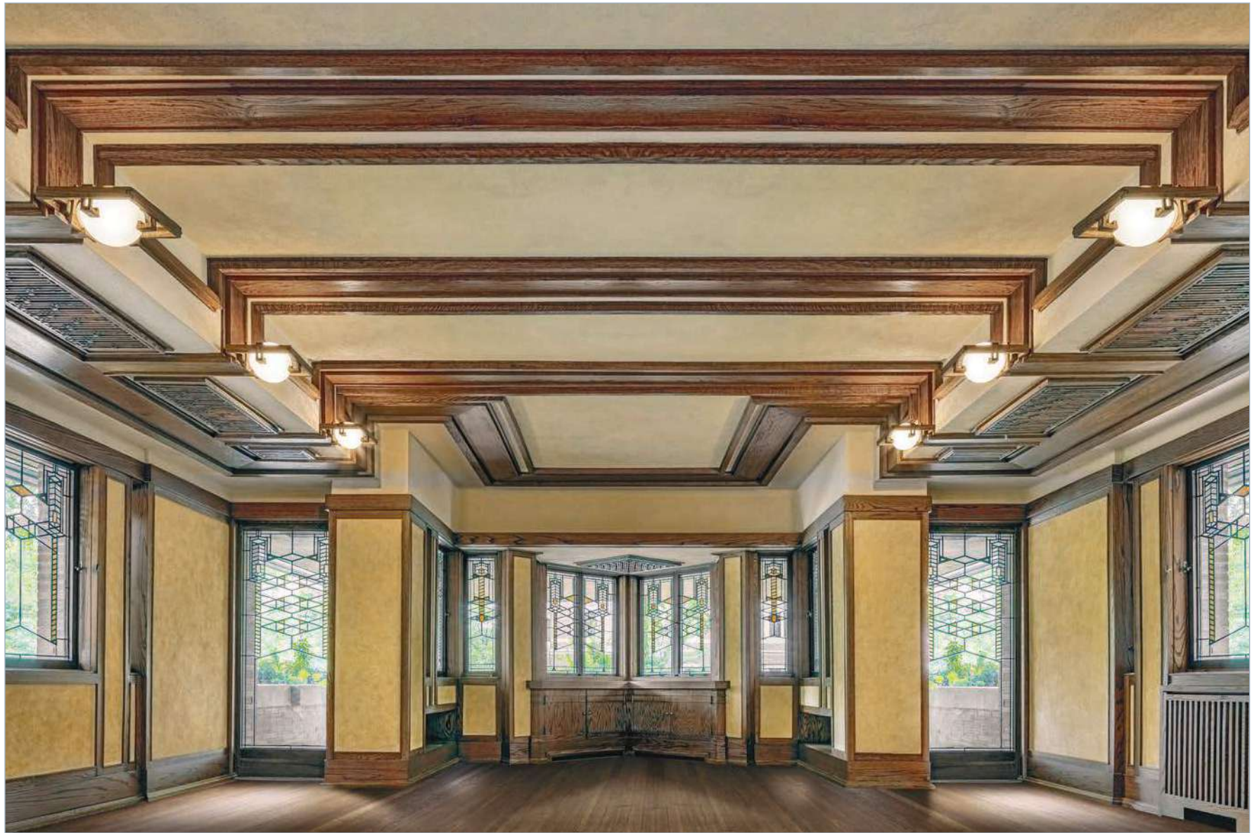
Robie House Living Room, view facing north showing prow feature of main level, wood striping of ceiling treatment, spherical sconce light fixtures, and art glass casement windows and porch doors.
